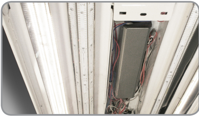
Figure 2: Integral LED Battery Packs install within, atop, or next to the LED fixture to provide emergency power. In this photo, a battery pack installs within the troffer to power the LED strips.
